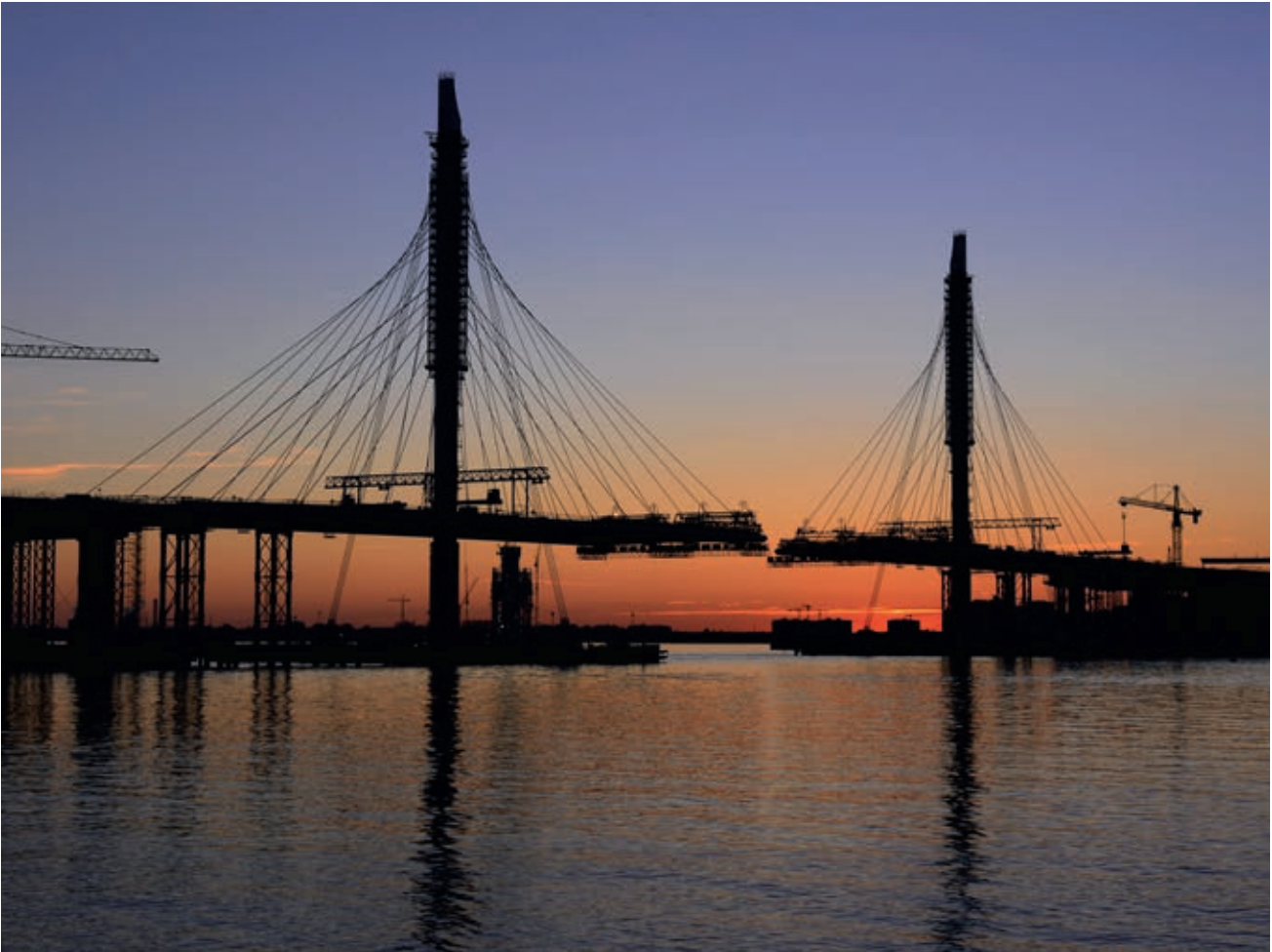
Russia, Western High Speed Diameter in St Petersburg.
