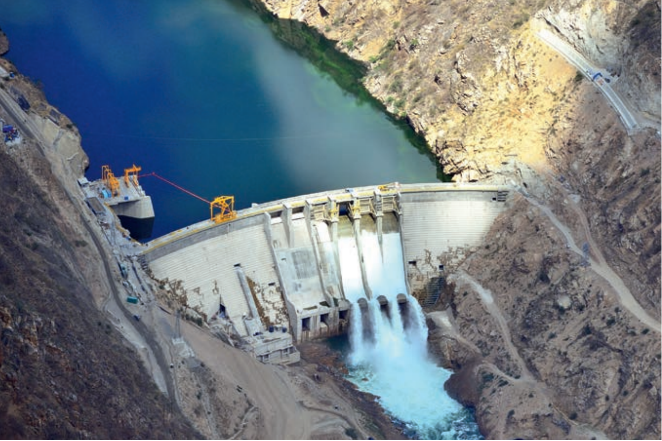
Peru, Cerro del Águila hydroelectric plant.
