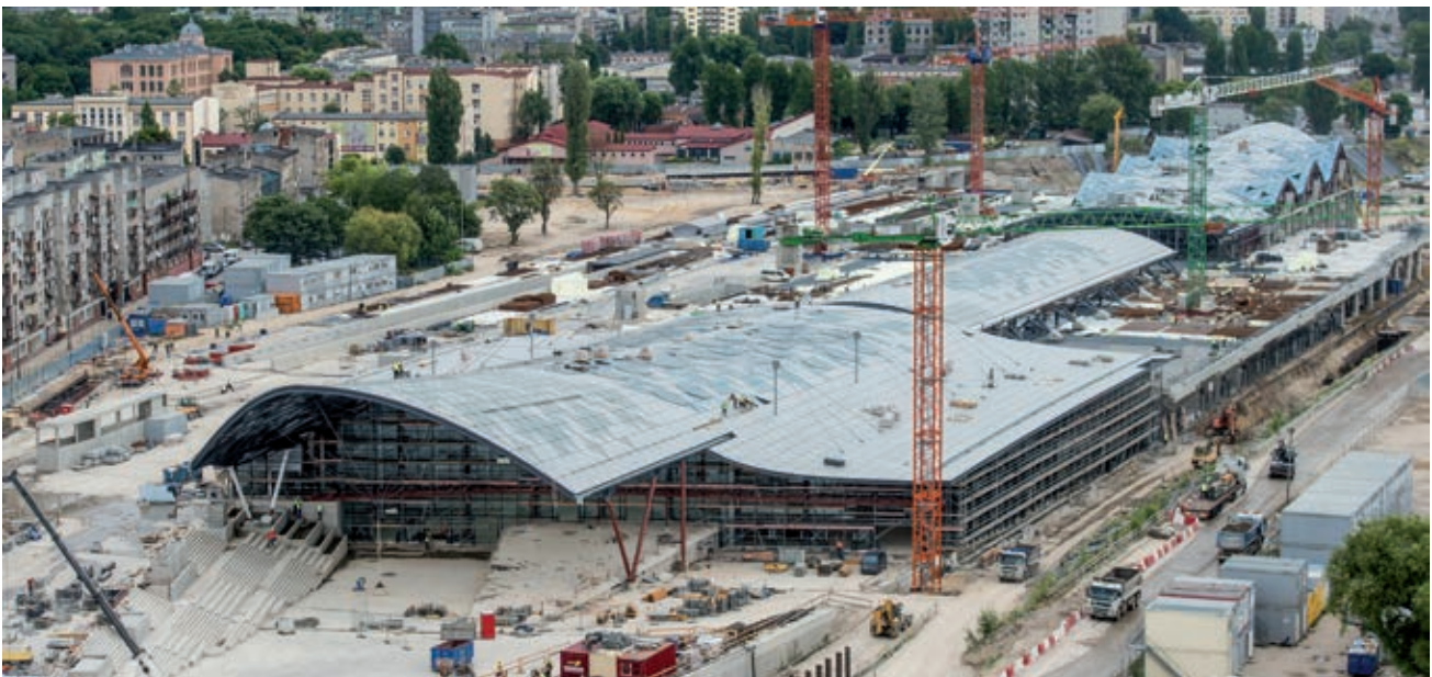
Poland, Łódź-Fabryczna railway project.
