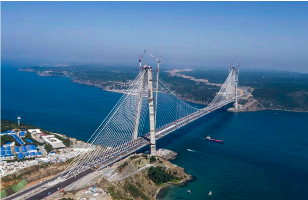
Turkey, Third Bridge on Bosphorus and North Marmara Highway.
