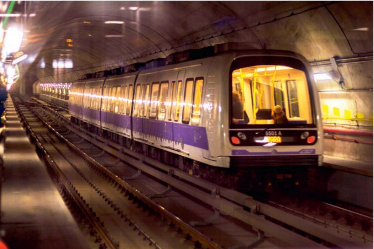
Italy, Milan Subway Line 5.
