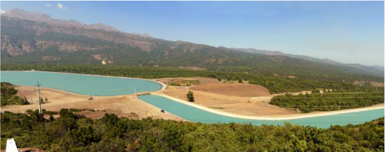
Chile, Chacayes Hydroelectric plant.
