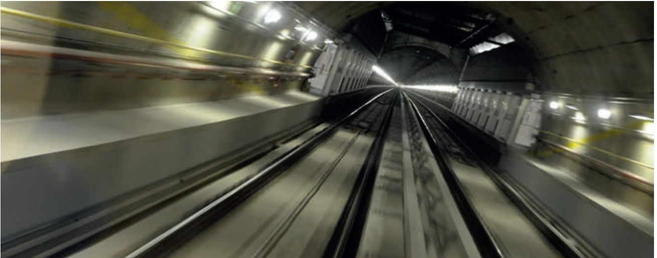
Italy, Milan Subway Line 5.
