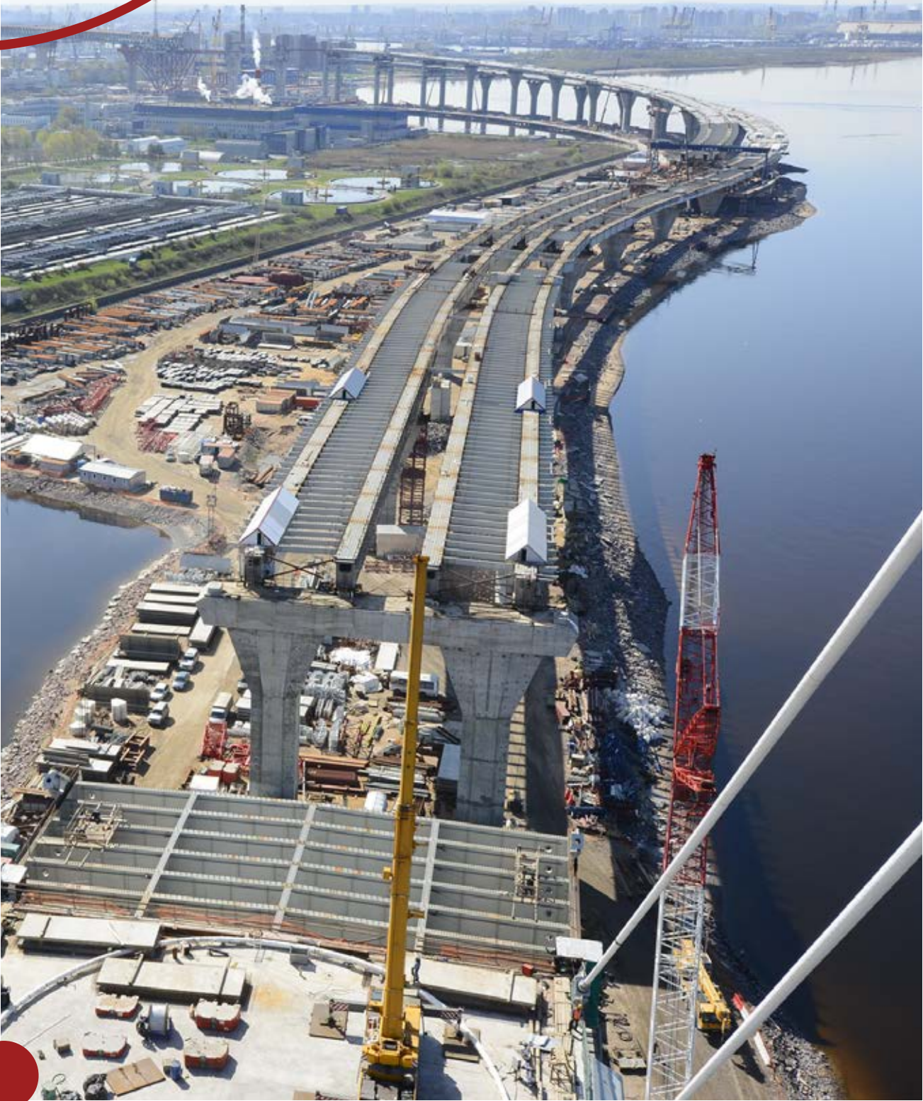
Russia, Western High Speed Diameter in St Petersburg.
