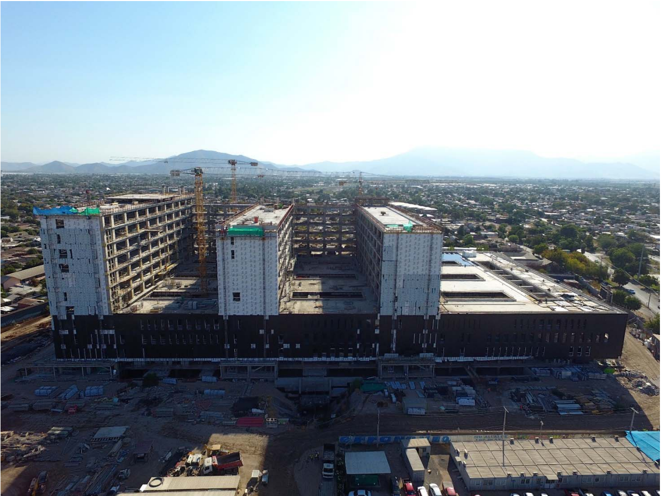
CHILE – West Metropolitan Hospital, Santiago.
