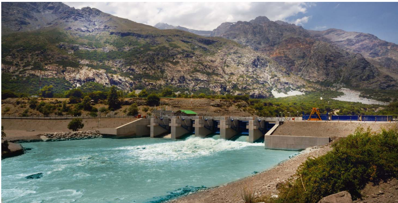
CHILE – Chacayes Hydroelectric Plant.
