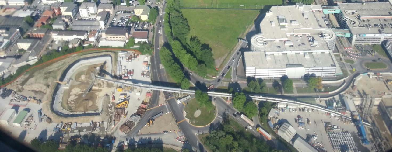
ITALY – Line 4 of Milan underground.
