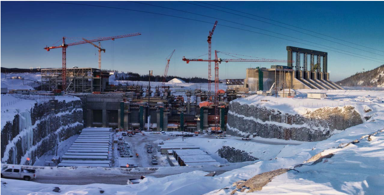
CANADA –Muskrat Falls Hydroelectric Project (© Alberto Audisio).
