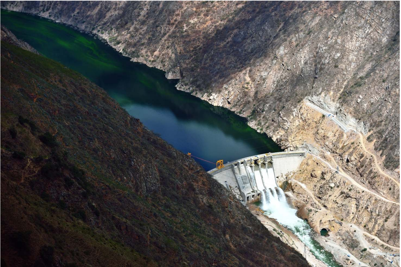
PERU –Cerro del Águila Hydroelectric Plant.
