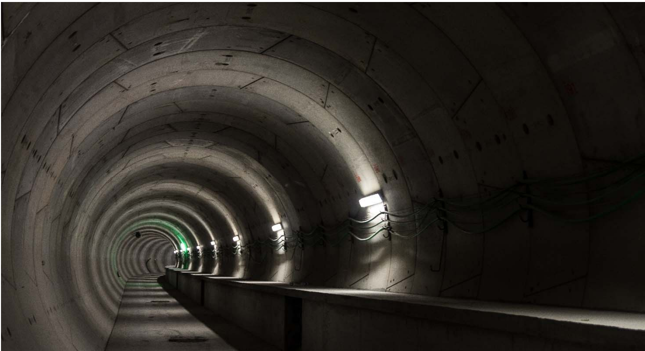
ITALY – Line 4 of Milan underground.
