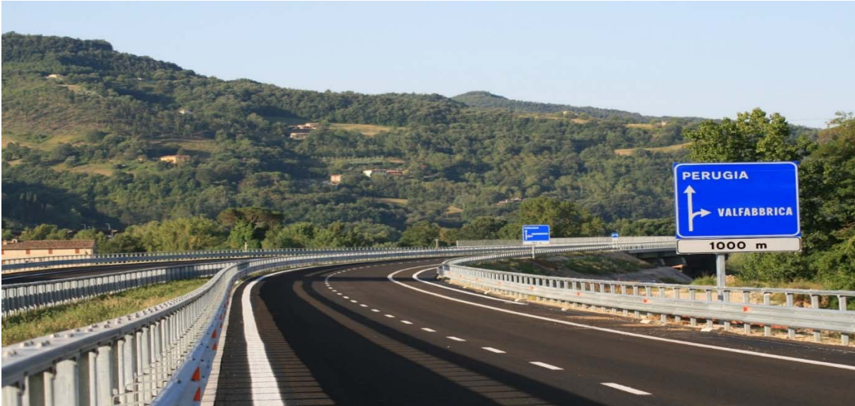
ITALY –Marche-Umbria Quadrilatero road network (Pianello-Valfabbrica section).
