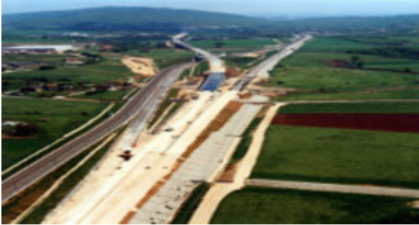
Rome-Naples High-Speed Railway | Location: Italy
