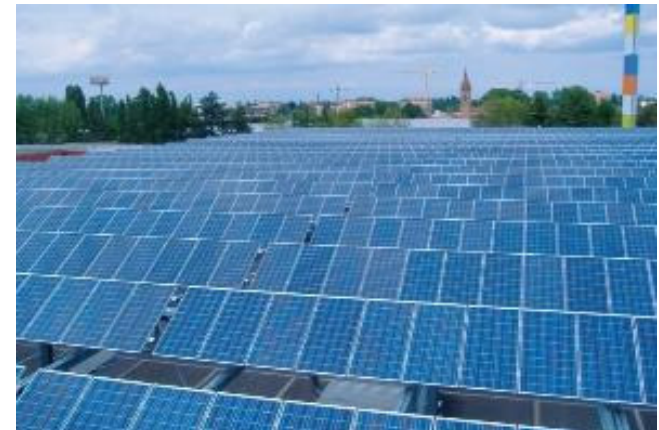
COOP Adriatica Photovoltaic plant | Location: Italy
