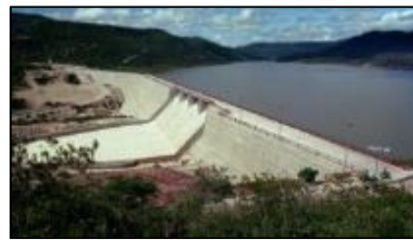
CONCEPCION HYDRO PROJECT | HONDURAS 1991 INGERSOLL-RAND ITALIA
