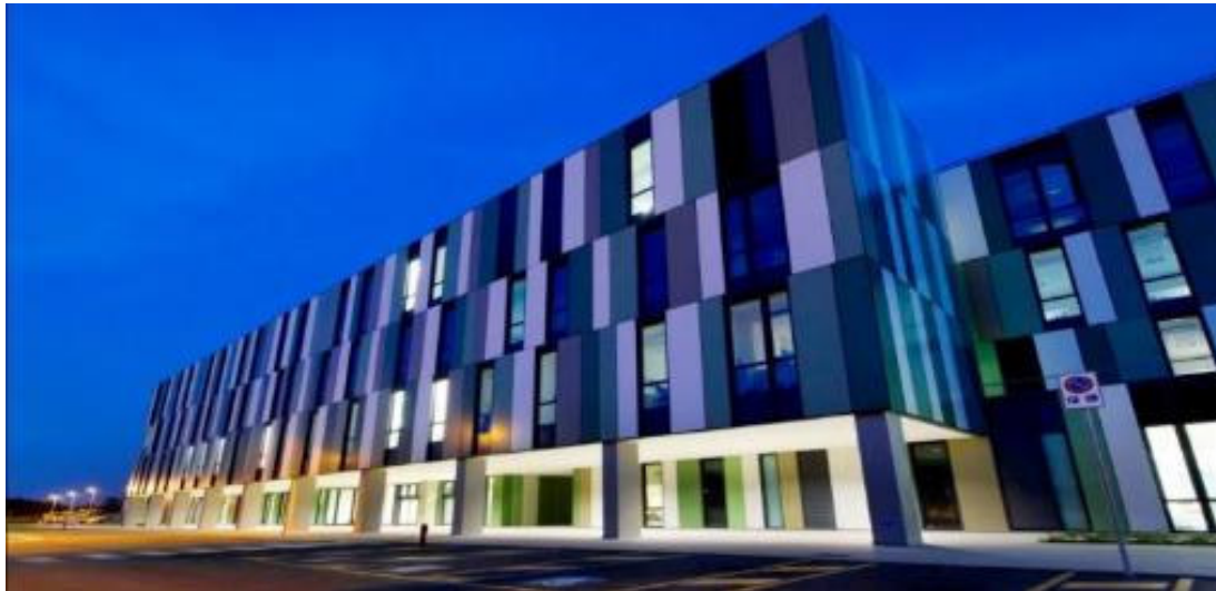
New Hospital in Pistoia ( Ospedale San Jacopo ) | Location: Italy | under management
