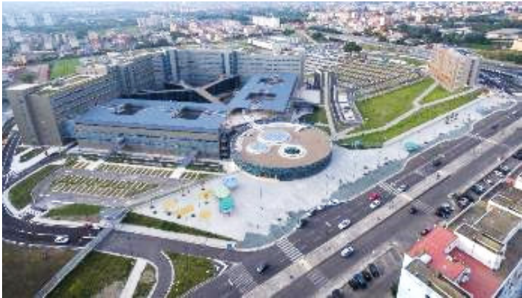
New Hospital In Naples | Location: Italy
