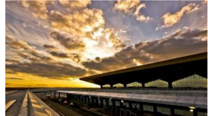
Pulkovo International Airport | Location: Russia, Saint Peterburg
