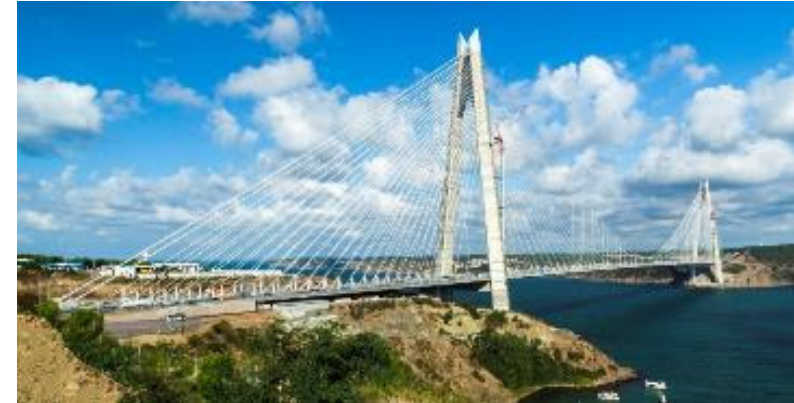
Northern Marmara Motorway and 3rd Bosphorus Bridge | Location: Turkey
