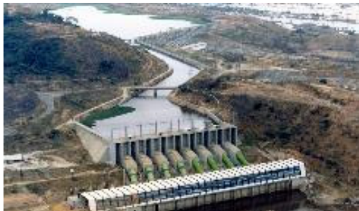
Inga Hydroelectric Project – phase 1 and phase 2 | Location: DR Congo
