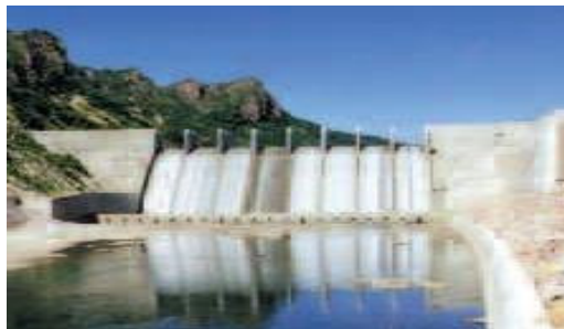
Nacaome Valley RCC Dam | Location: Honduras
