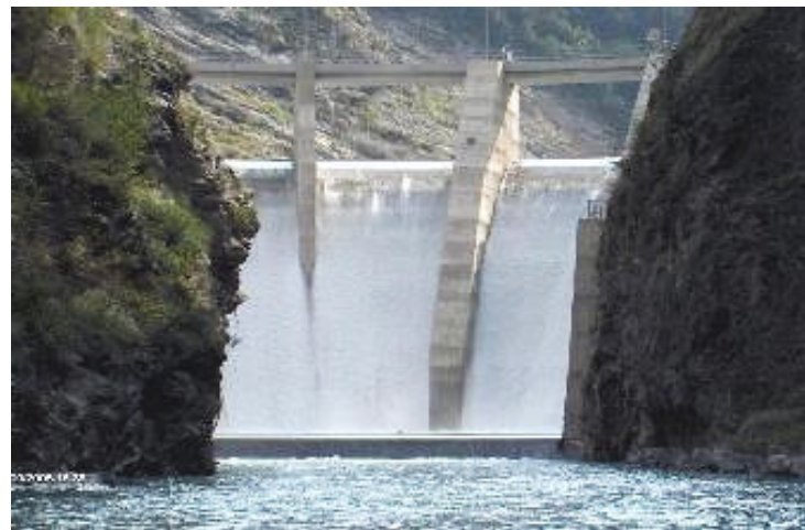
Pont Ventoux Hydroelectric Power Plant | Location: Italy
