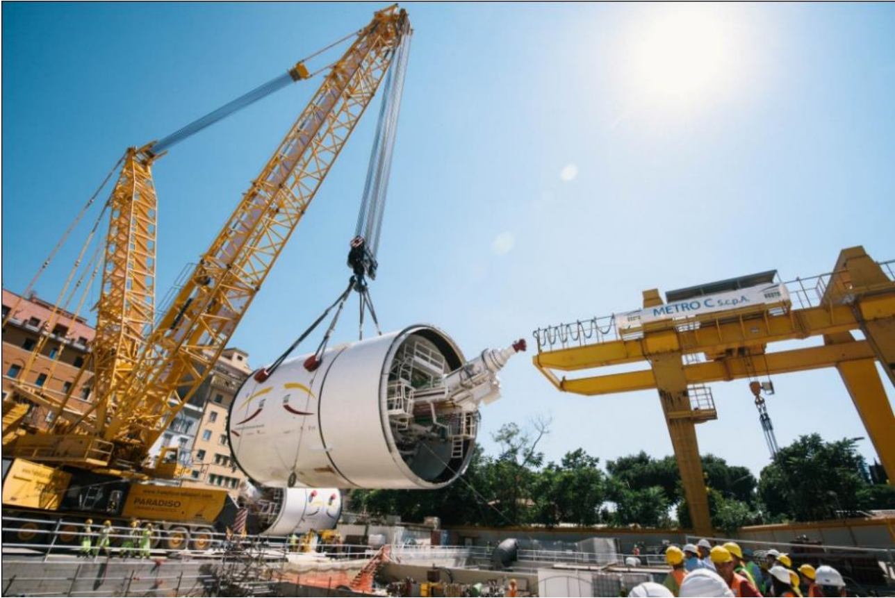
Line C, Rome Underground - Italy | 3.3 Shaft Site, TBM launch – Photo: Metro C.
