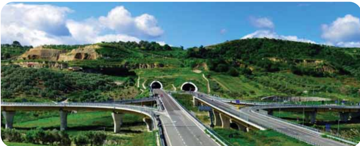
NR-106 state road Jonica (Lot DG-41), Italy | Render Avena Viaduct – Credits: Astaldi Archives
