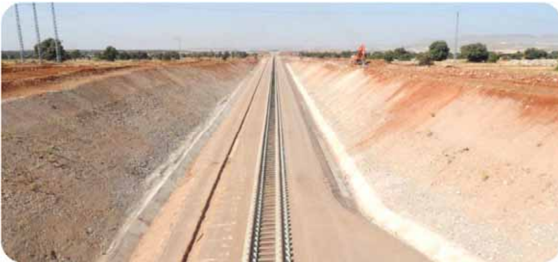
Saida - Tiaret railway line (Algeria) – Credits: Astaldi Archives
