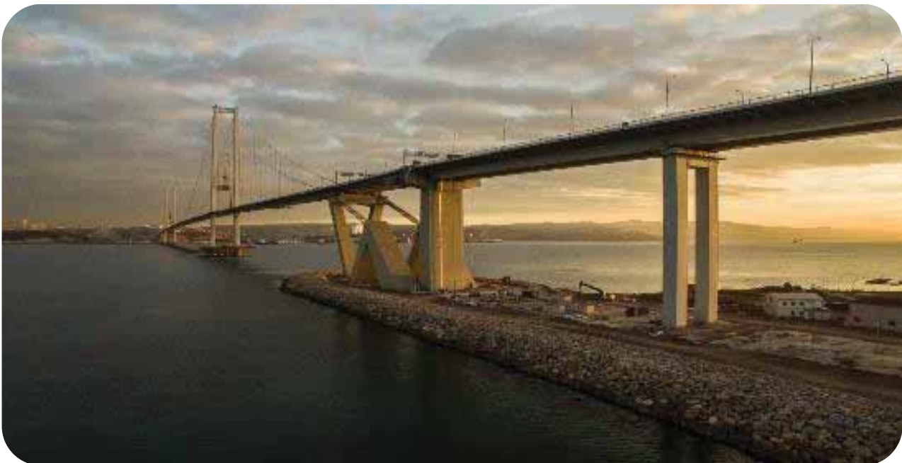
Gebze-Orhangazi-Izmir motorway, Turkey | Izmit Bay Bridge – Credits: Astaldi Archives
