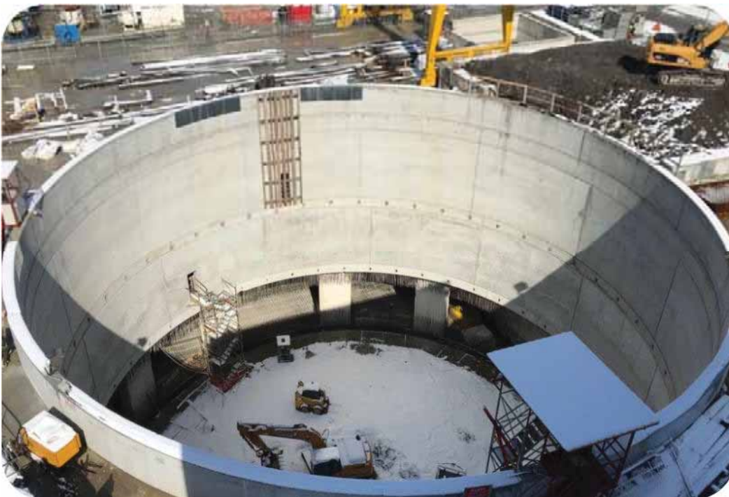
Line 1 of the Naples Metro, Capodichino Station | Work site – Credits: Astaldi Archives
