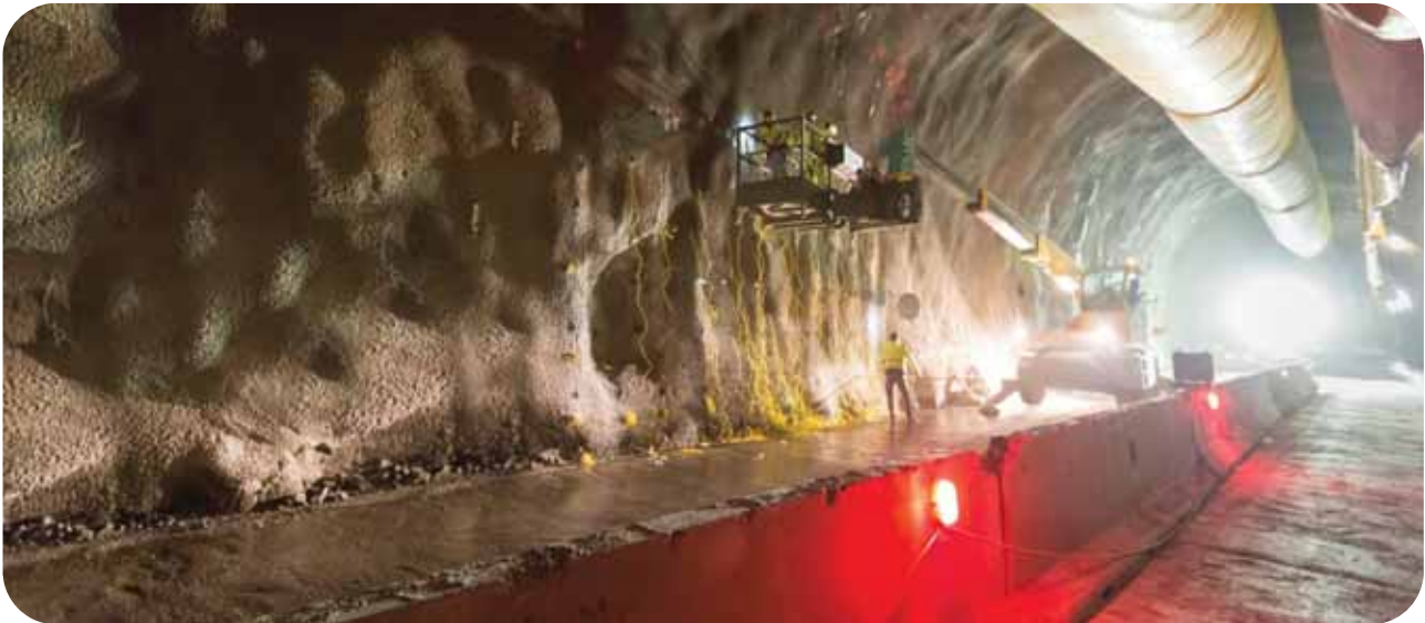
Brenner Base Tunnel, Italy | Lot "Mules 2-3" work site. – Credits: BBT-SE.
