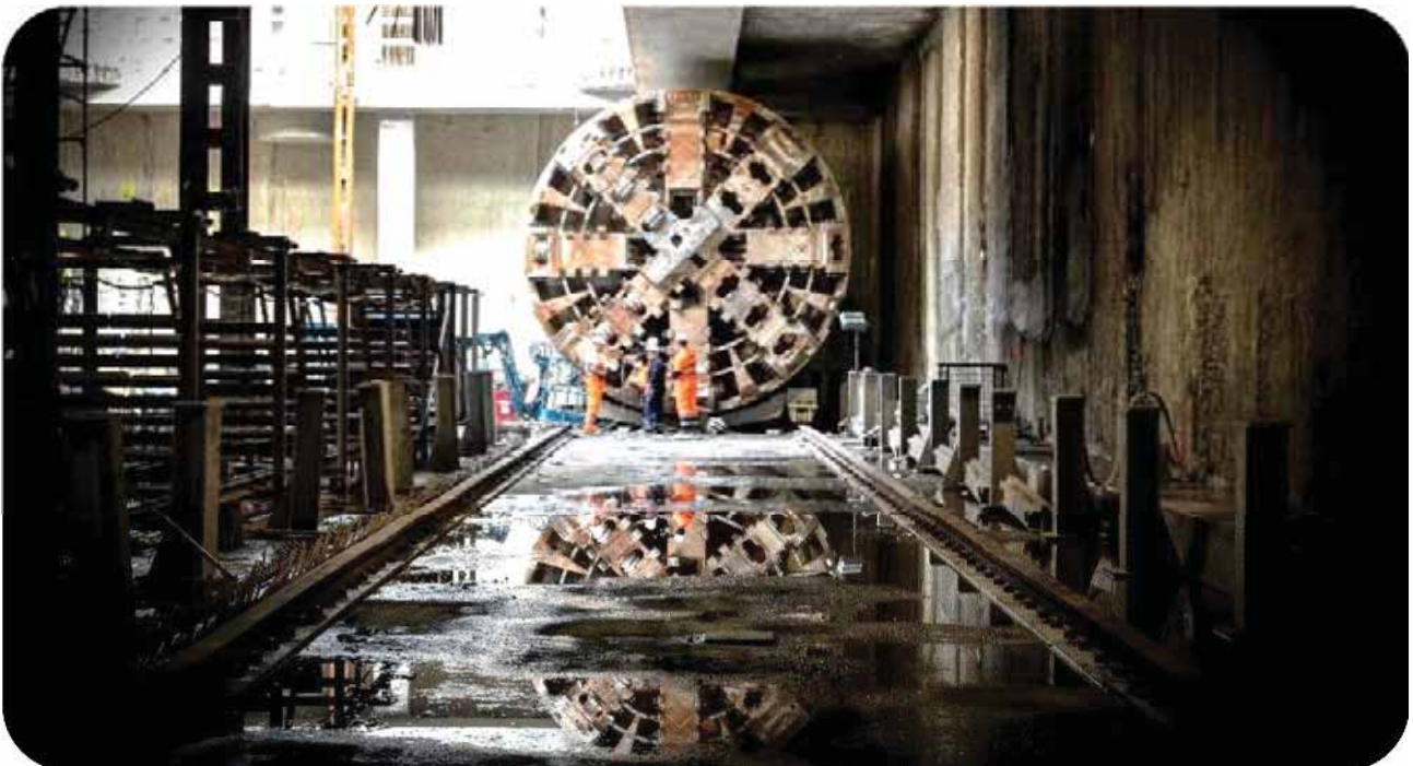
Line 2 of the Warsaw metro (Phase 2), Poland | TBM crossing – Credits: Astaldi Archives
