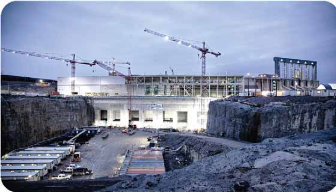
Muskrat Falls hydroelectric project (Canada) | View from the river bank – Credits: Astaldi Archives
