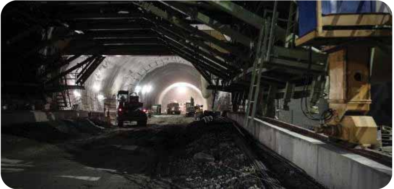
S-7 Expressway, Poland – Credits: Astaldi Archives
