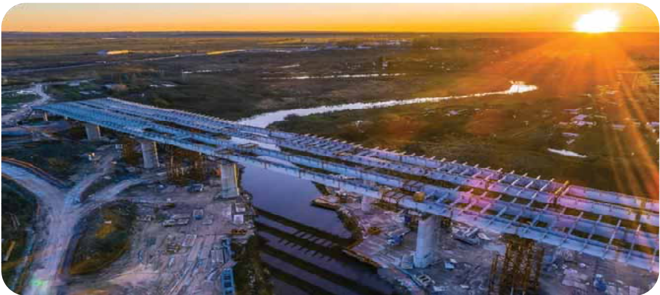
Moscow-St. Petersburg M-11 motorway (Russia) - Credits: Astaldi Archives
