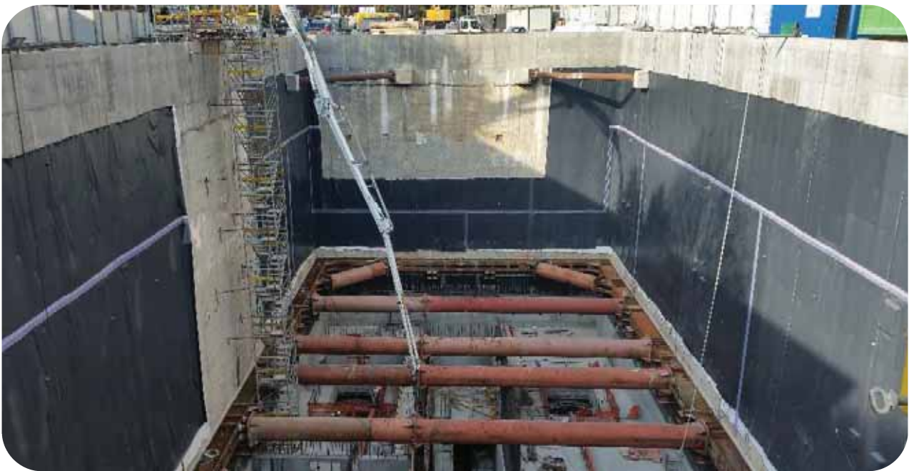
Line 4 of the Milan metro, Italy | Dateo Station work site – Credits: Astaldi Archives
