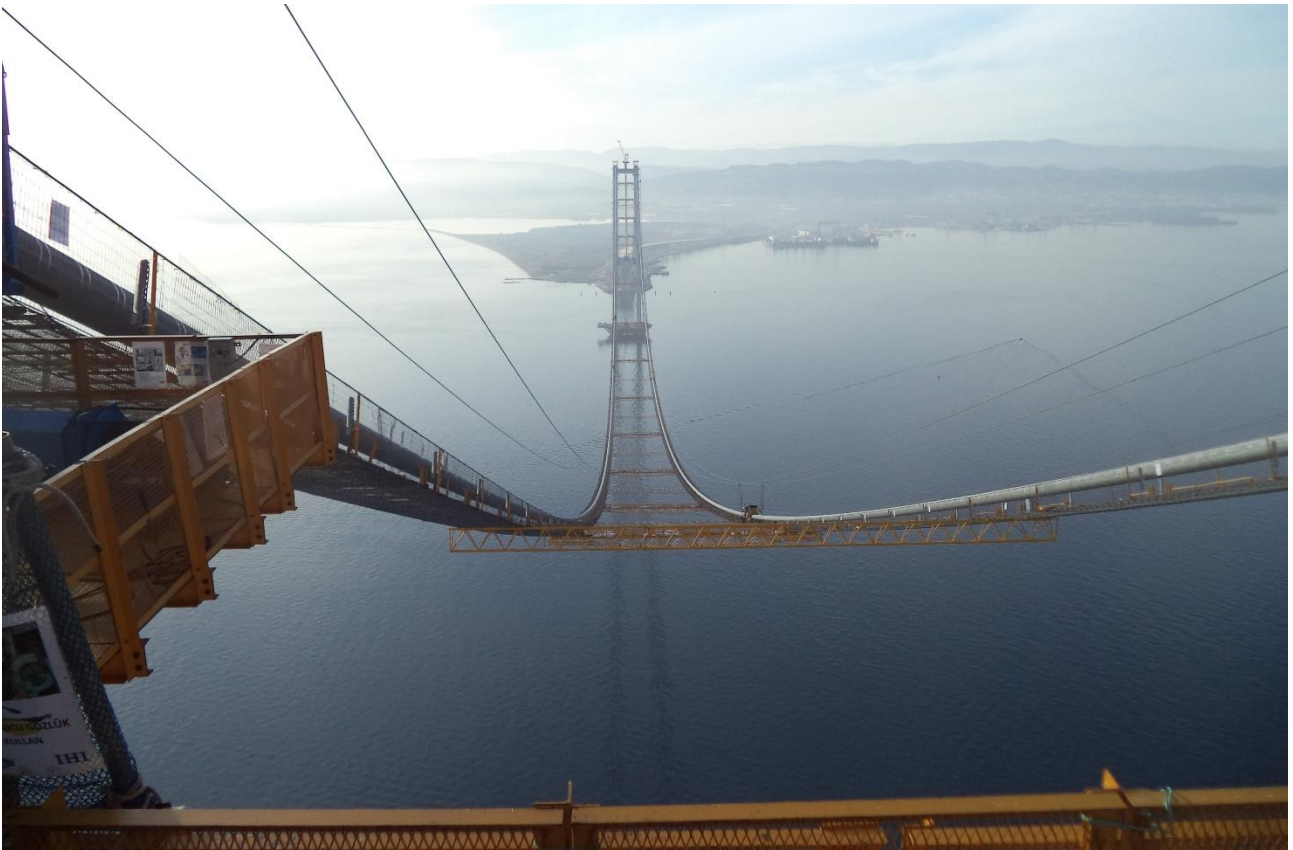
TURKEY, GEBZE-ORHANGAZI-IZMIR MOTORWAY (Izmit Bay Bridge) – This is the fourth suspension bridge in the world.
