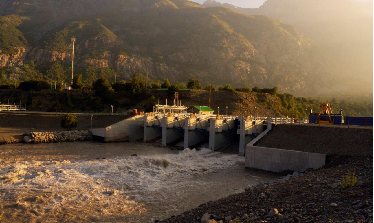
CHACAYES HYDROELECTRIC PLANT – The 1 st totally eco-compatible plant built in Chile
