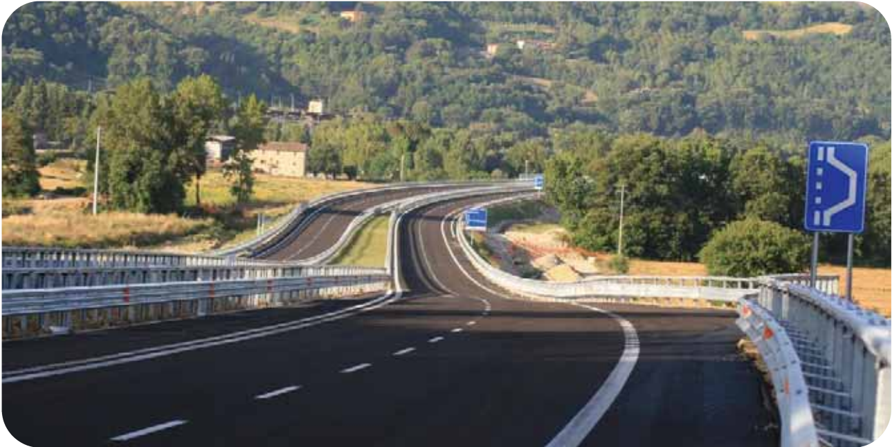
Quadrilatero Marche-Umbria road system (maxi lot 2), Italy | Completion of the road system – Credits: Astaldi Archives
