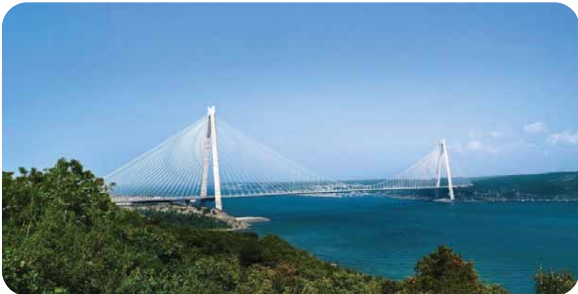
Northern Marmara Highway Project, (Turkey) | Third Bosphorus Bridge – Credits: Astaldi Archives
