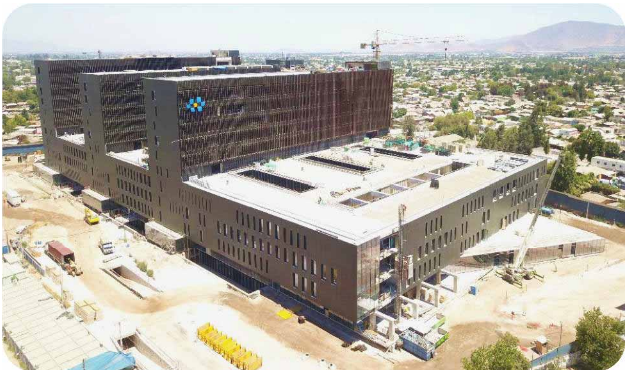
West Metropolitan Hospital in Santiago (Chile) | Aerial view – Credits: Astaldi Archives
