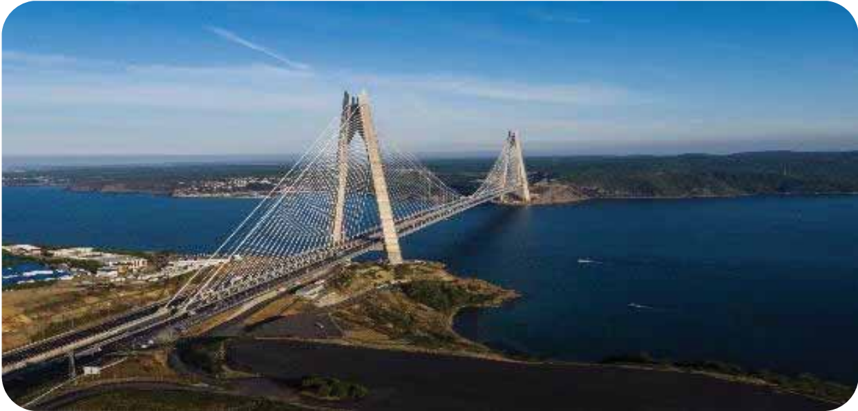
Northern Marmara Highway Project, Turkey | Third Bosphorus Bridge – Credits: Astaldi Archives
