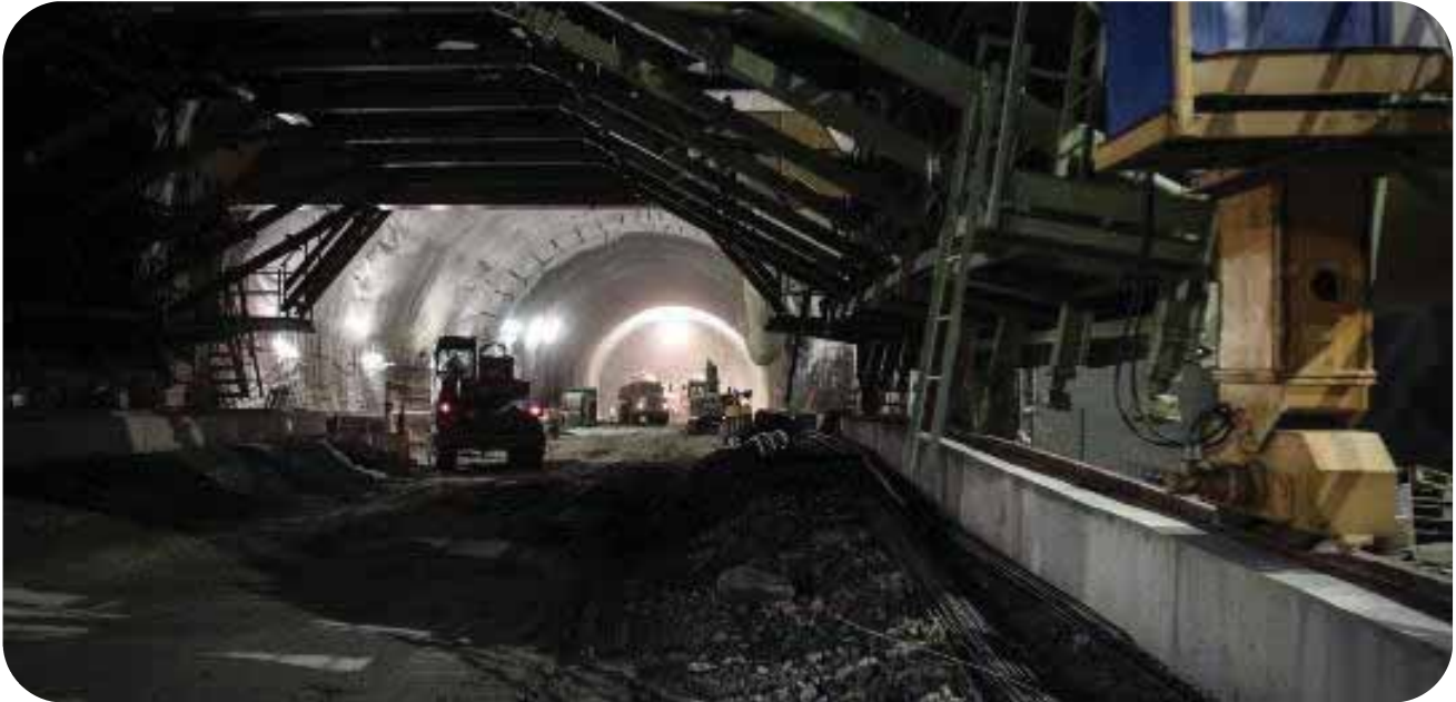
S-7 Expressway, Poland – Credits: Astaldi Archives
