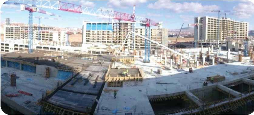
Etlik Integrated Health Campus, Ankara, Turkey | Work site – Credits: Astaldi Archives
