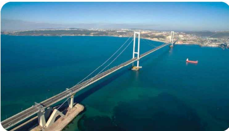
Gebze-Orhangazi-Izmir motorway (Turkey) | Izmit Bay Bridge – Credits: Astaldi Archives
