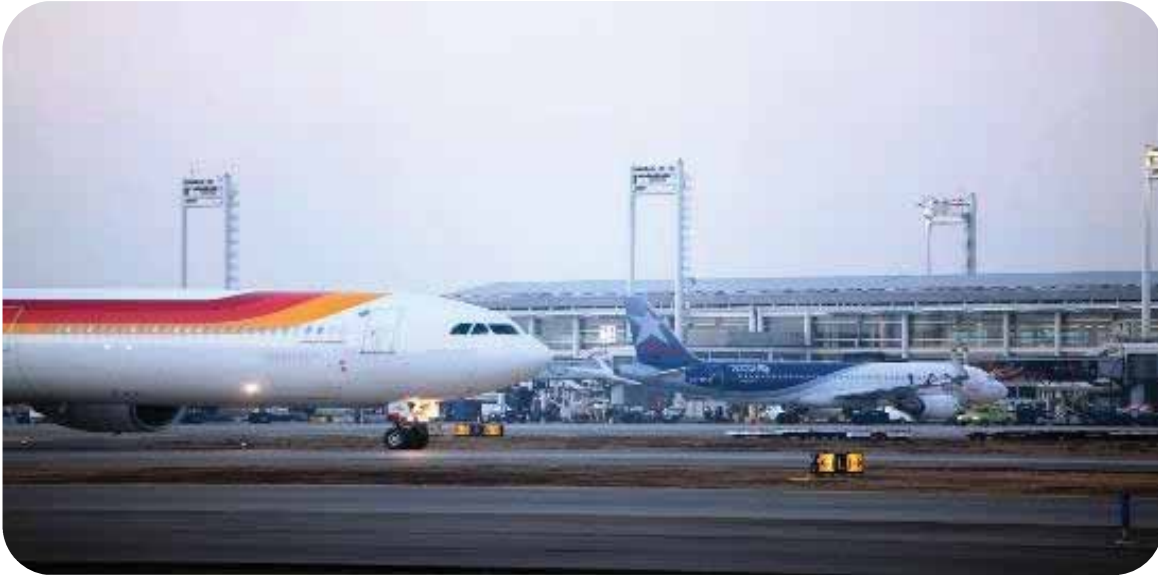
Arturo Merino Benítez International Airport, Chile | Exterior – Credits: Astaldi Archives
