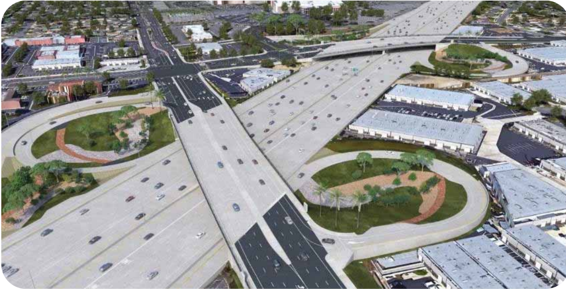
Interstate I-405 to Los Angeles (California), USA | View from above ( render ) – Credits: Astaldi Archives
