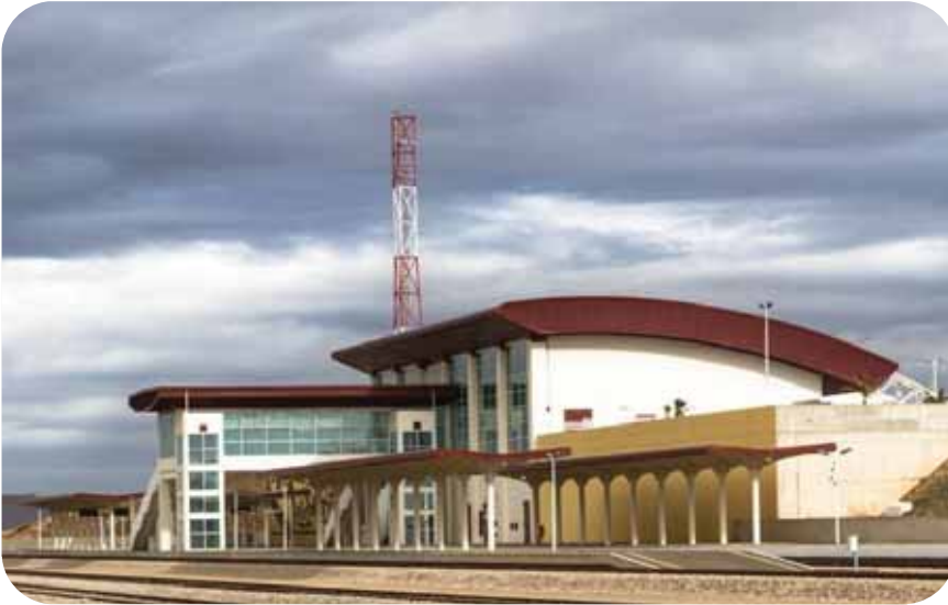
Saida-Moulay Slissen railway line (Algeria) – Credits: Astaldi Archives
