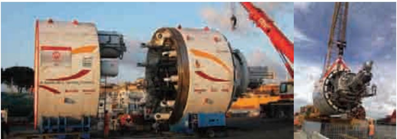
Putting into operation of the first TBM to be used to construct the new Line C of the Rome underground.
