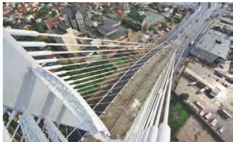
Romania, Basarab Overpass.
