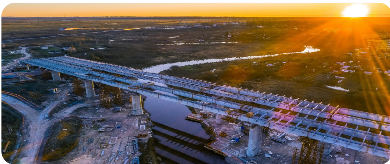
Moscow-St. Petersburg M-11 motorway (Russia) - Credits: Astaldi Archives
