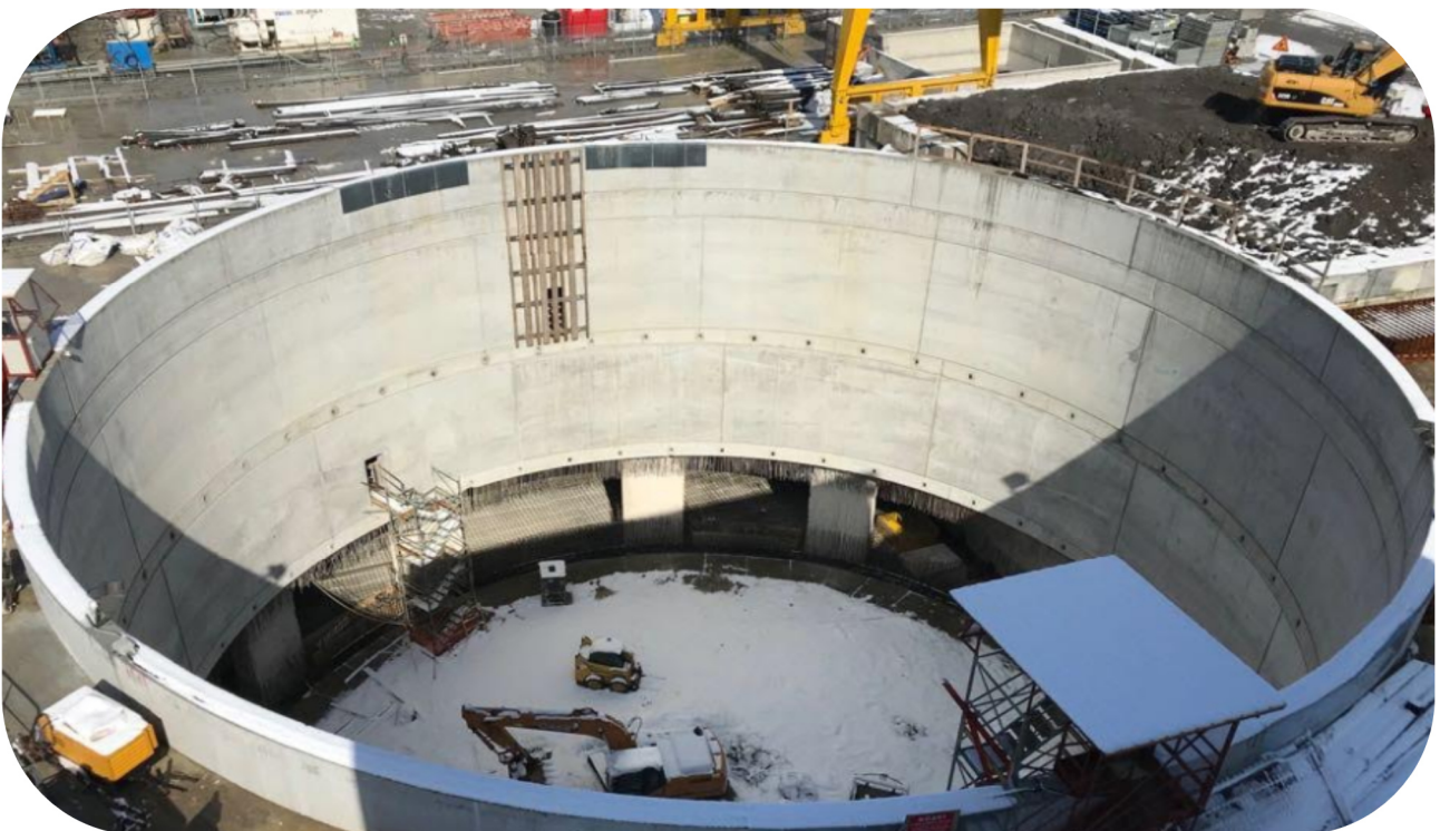
Line 1 of the Naples Metro, Capodichino Station | Work site – Credits: Astaldi Archives
