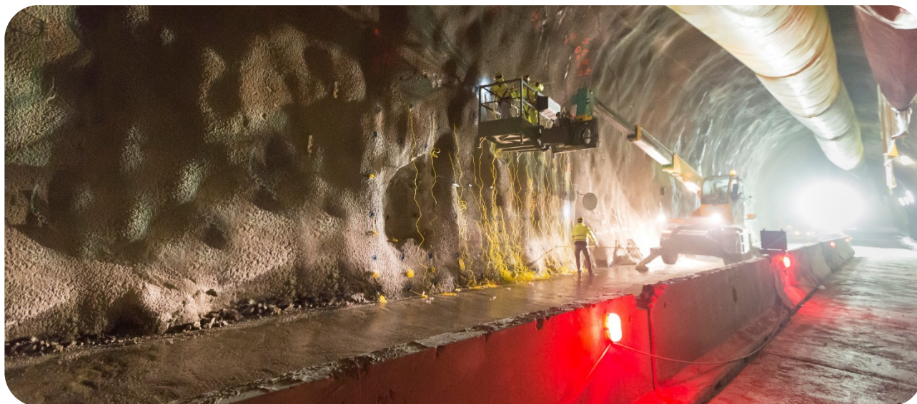
Brenner Base Tunnel, Italy | Lot "Mules 2-3" work site. – Credits: BBT-SE.
