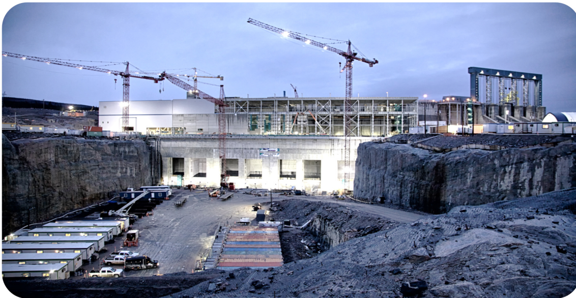
Muskrat Falls hydroelectric project (Canada) | View from the river bank – Credits: Astaldi Archives
