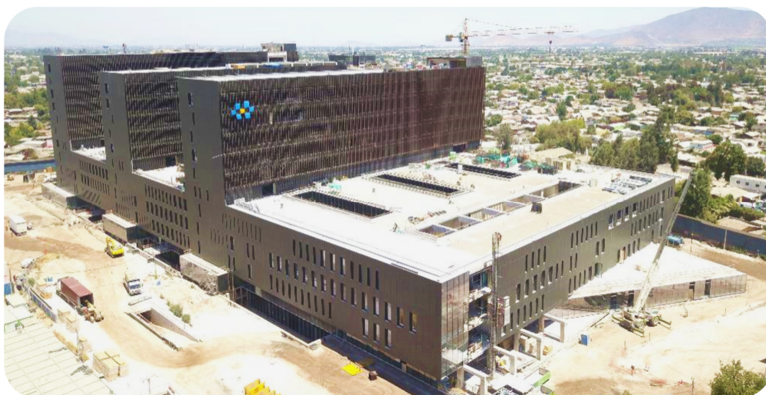
West Metropolitan Hospital in Santiago (Chile) | Aerial view – Credits: Astaldi Archives
