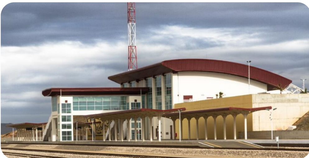
Saida-Moulay Slissen railway line (Algeria) – Credits: Astaldi Archives
