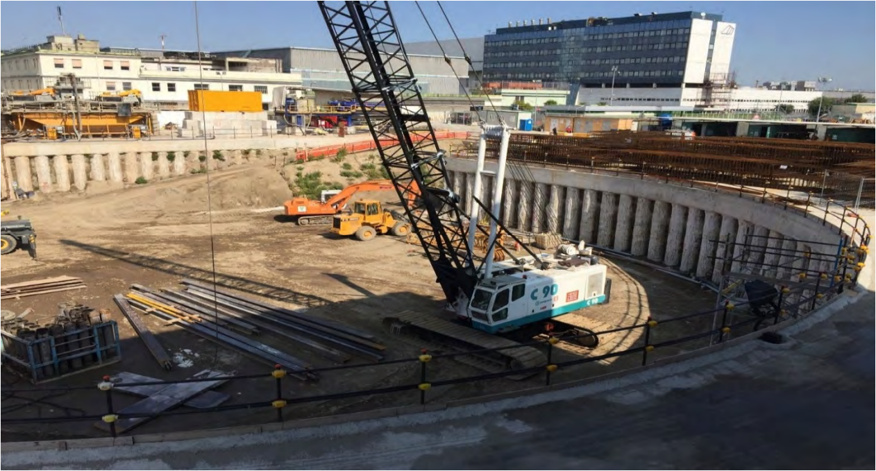
ITALY – Line 1 of Naples underground (Capodichino Station)
