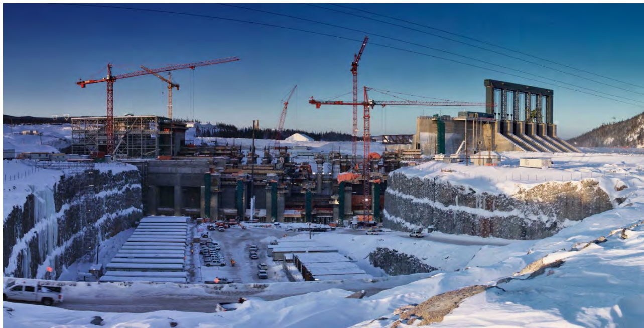
CANADA –Muskrat Falls Hydroelectric Project (© Alberto Audisio).
