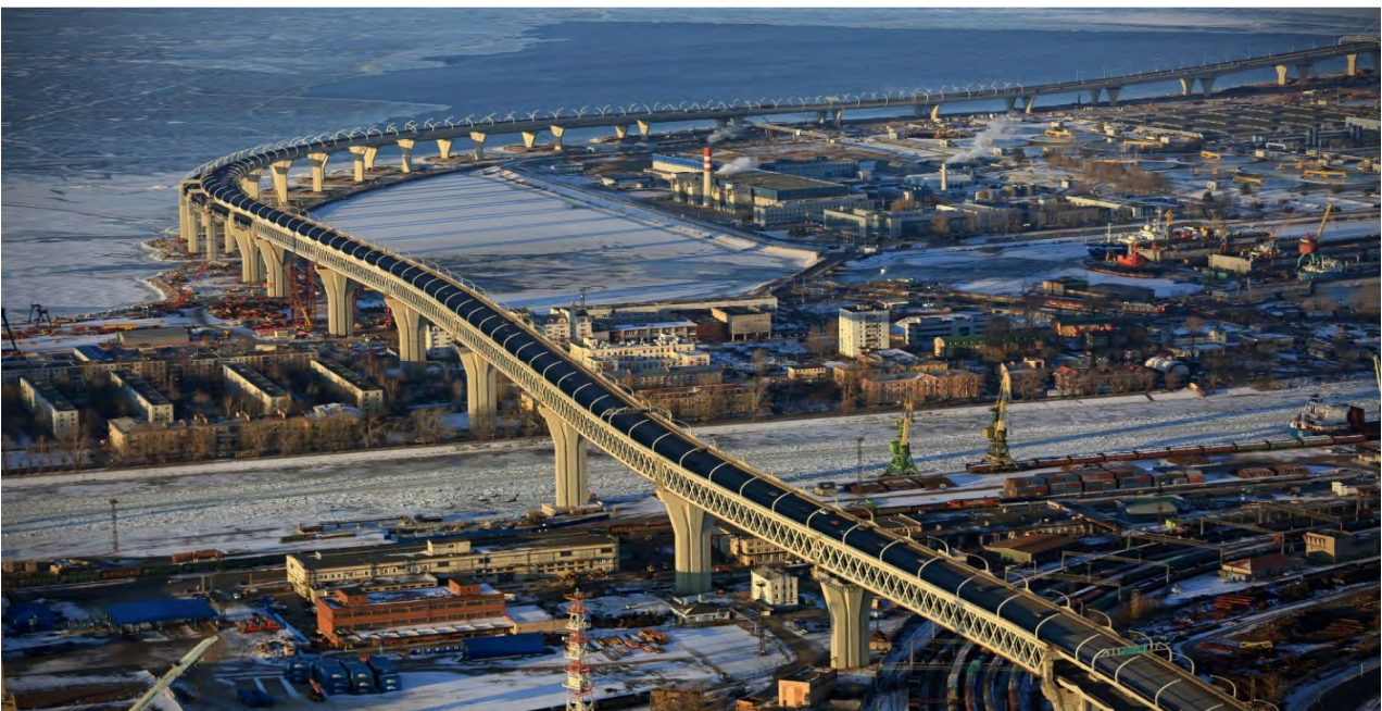
RUSSIA – Western High Speed Diameter in St. Petersburg.
