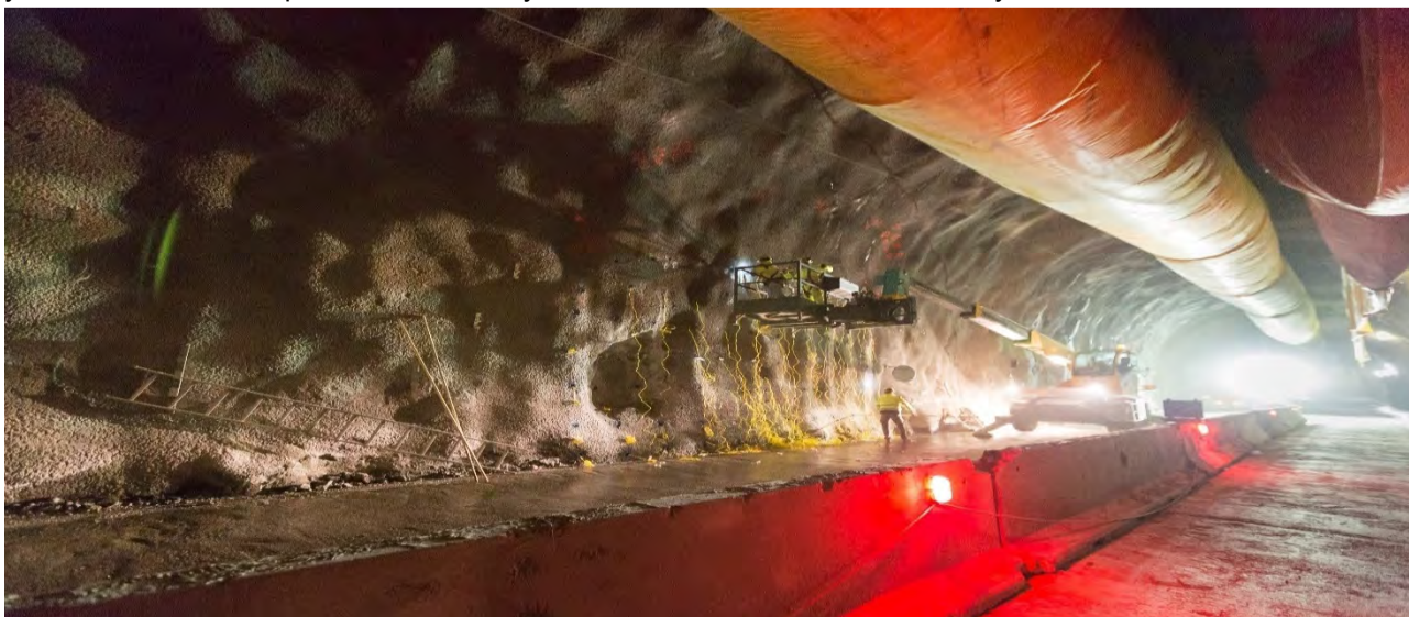
ITALY – Brenner Base Tunnel (drilling and blasting in December 2016).
