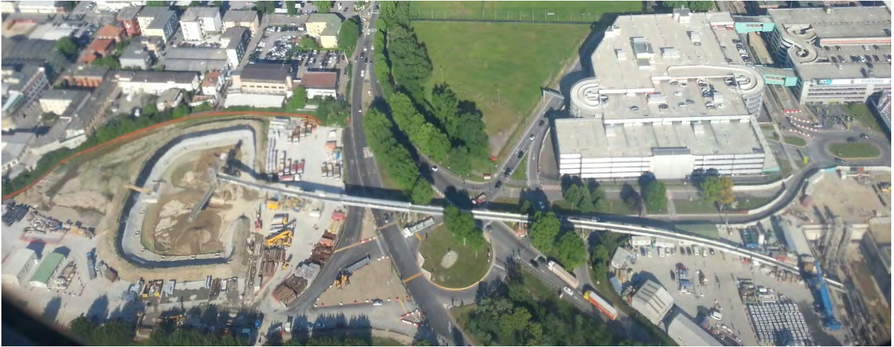
ITALY – Line 4 of Milan underground.
