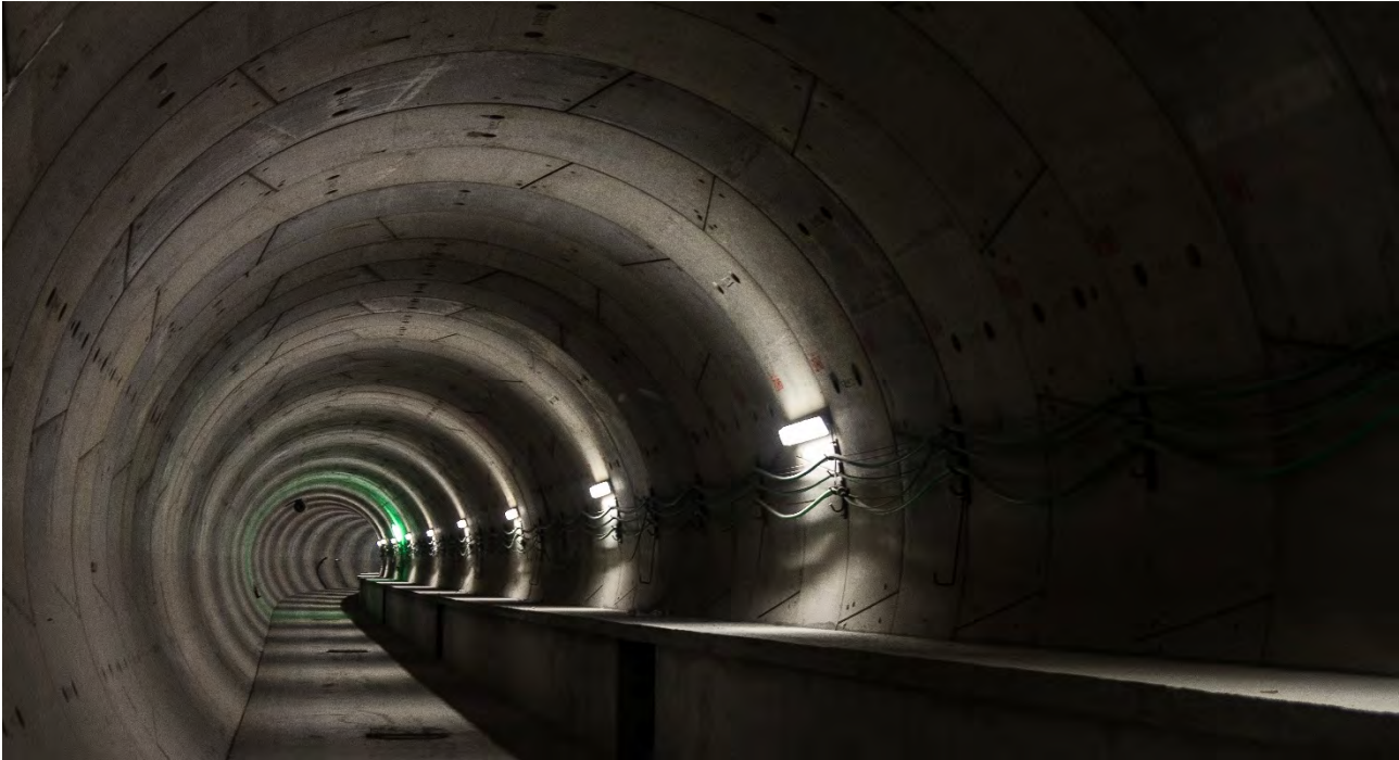
ITALY – Line 4 of Milan underground.
