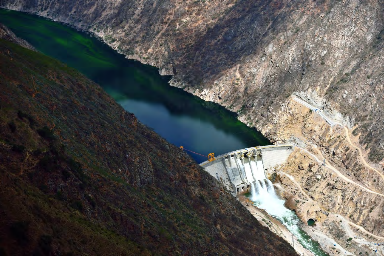
PERU –Cerro del Águila Hydroelectric Plant.
