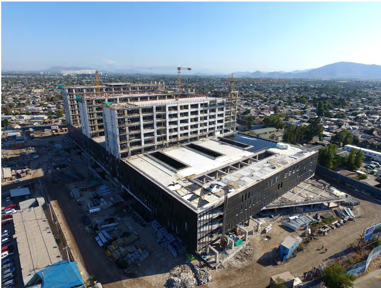
CHILE – West Metropolitan Hospital in Santiago.
