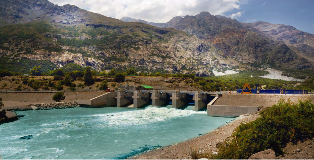
CHILE – Chacayes Hydroelectric Plant.
