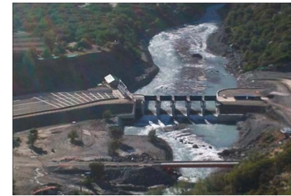
CHILE, Chacayes Hydroelectric Plant
