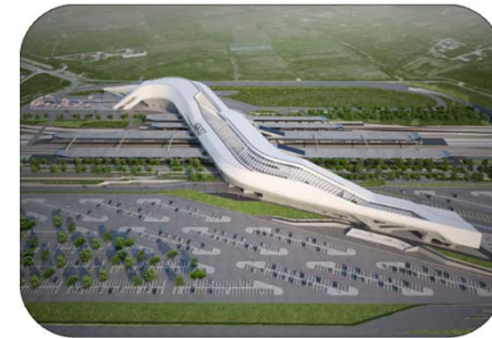
Naples-Afragola H-S railway station (construction) | Italy
