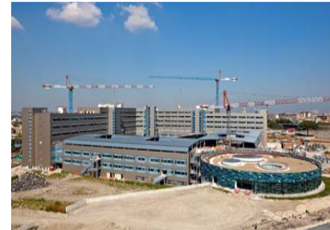
New Hospital in Naples | Italy
