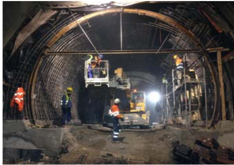
Warsaw Subway Line 2 | Poland
