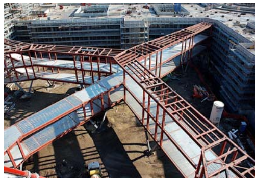
New Hospital in Naples | Italy
