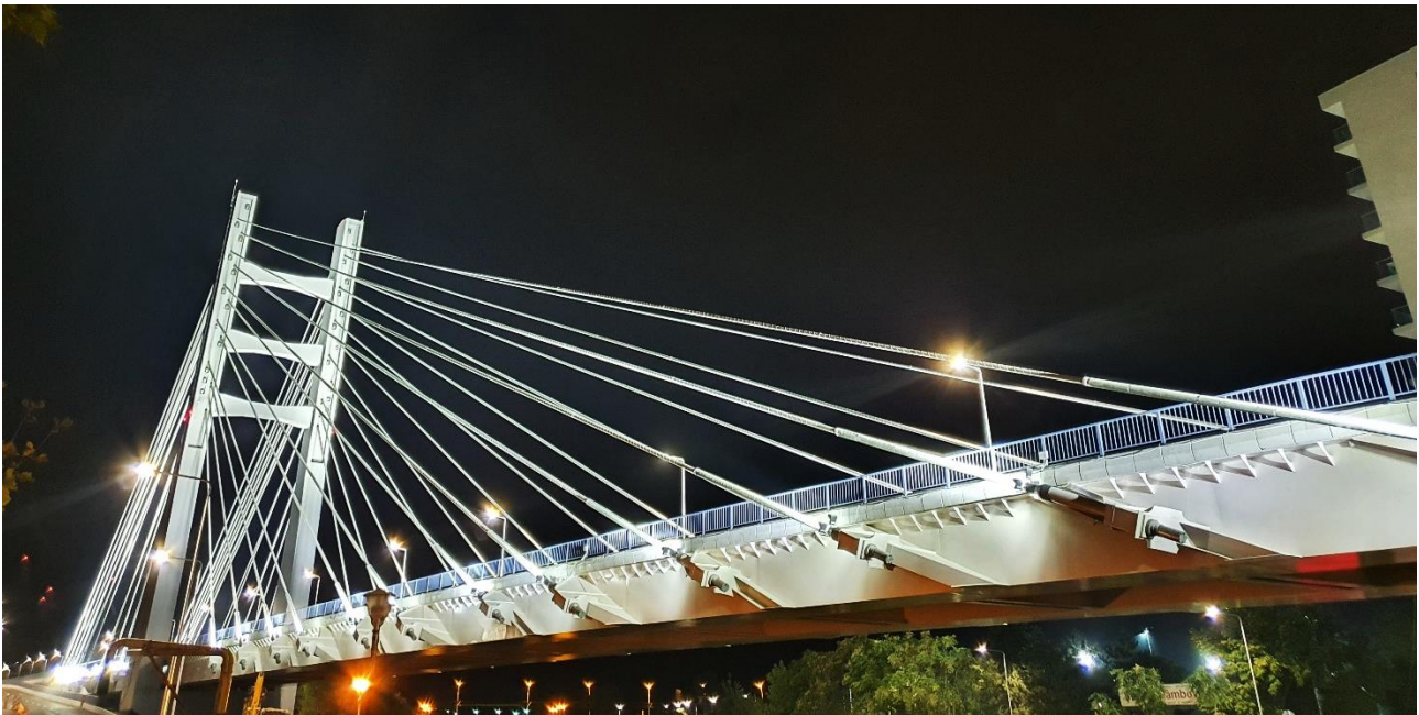
Cable-stayed bridge of Ciurel Overpass, Bucharest, Romania.
