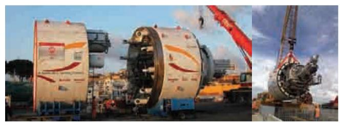
Putting into operation of the first TBM to be used to construct the new Line  ${\tt C}$  of the Rome underground.
