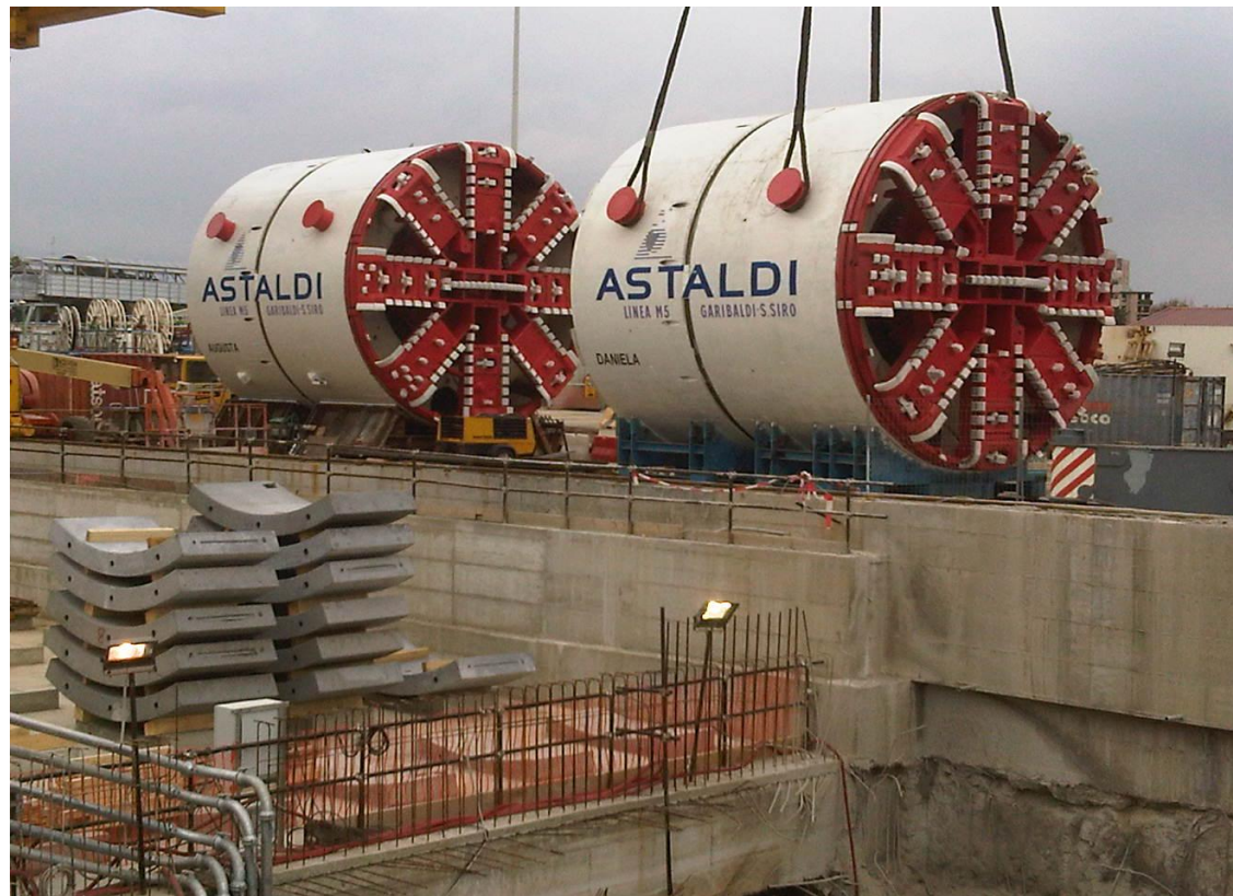
March 2012 - Lowering of TBM "Daniela" at sites for the extension of Line 5 of the Milan underground (Italy)
